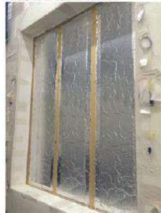
Photo 10 all boards installed
